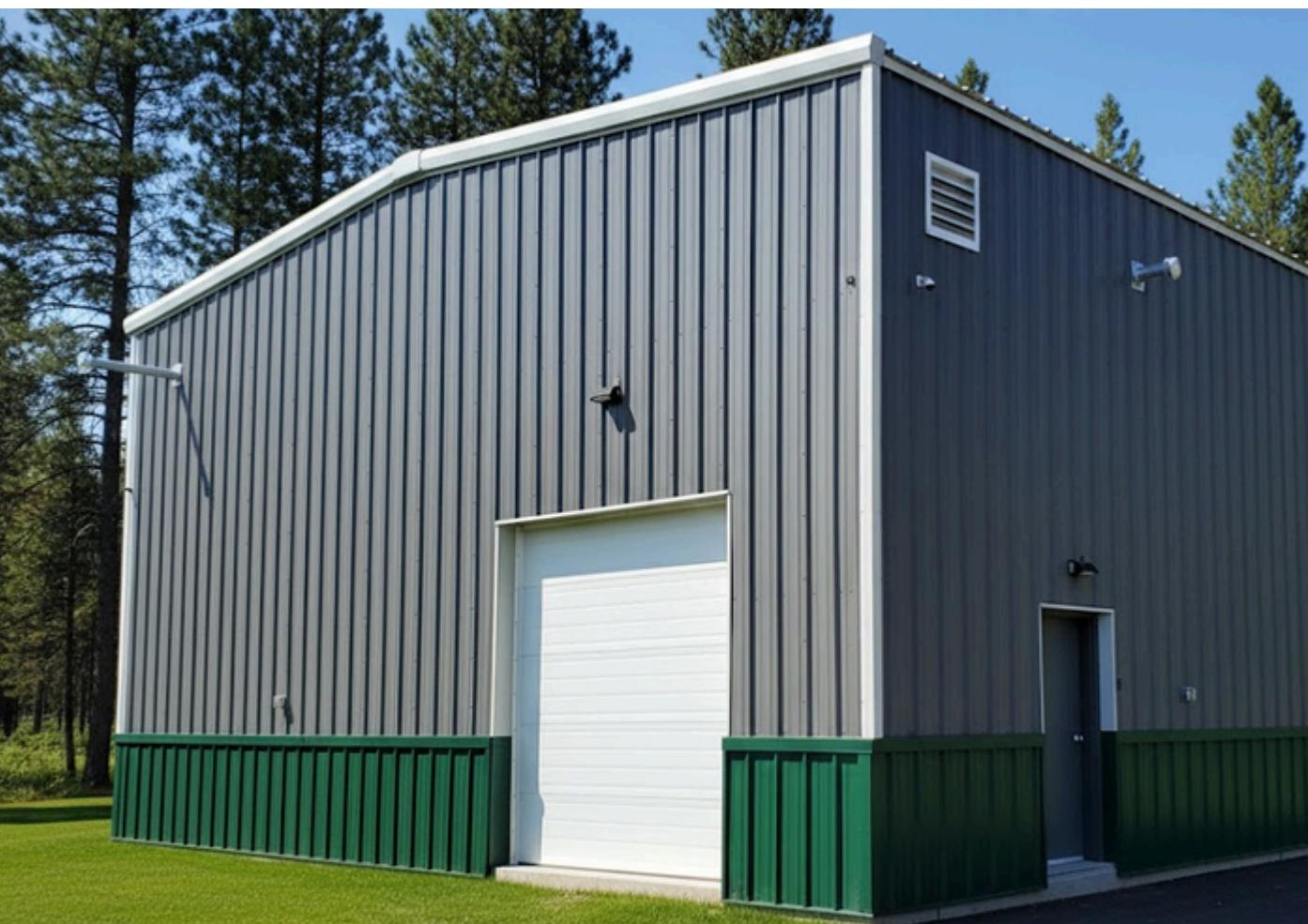
J trim and base trim are included with your building package to ensure a finished appearance and added protection against leaks and the possibility of rodent or insect infestation. Foam closures further ensure against leaks at the door openings. Jamb and header covers are used around door openings to complete the trim package.
