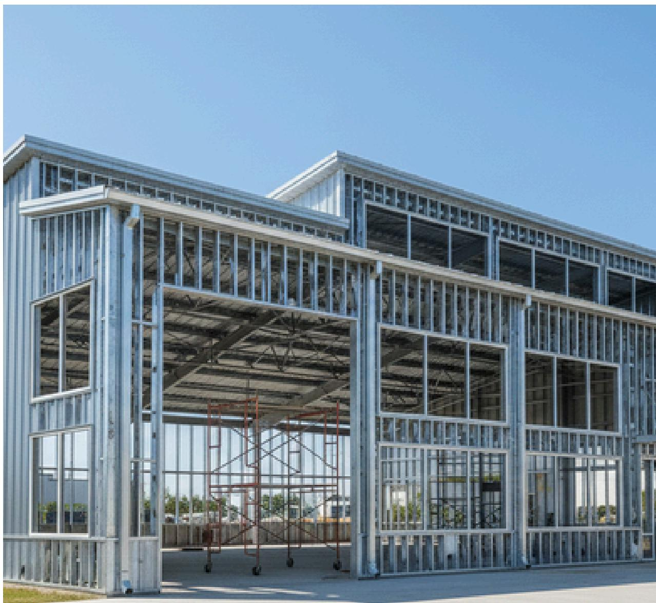
Our buildings come with a standardized hot-dip galvanized steel frame. All primary and secondary framing members are zinc coated and always outperform inferior paint primers used by other manufacturers. Our zinc galvanizing process prevents rust and increases the building's overall lifespan.
